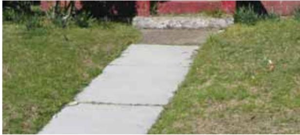
A resurfaced or repaired walkway shown here illustrates the contrast between the warm tones and rough texture of the old concrete and the new gray smooth concrete lacking aggregate.
